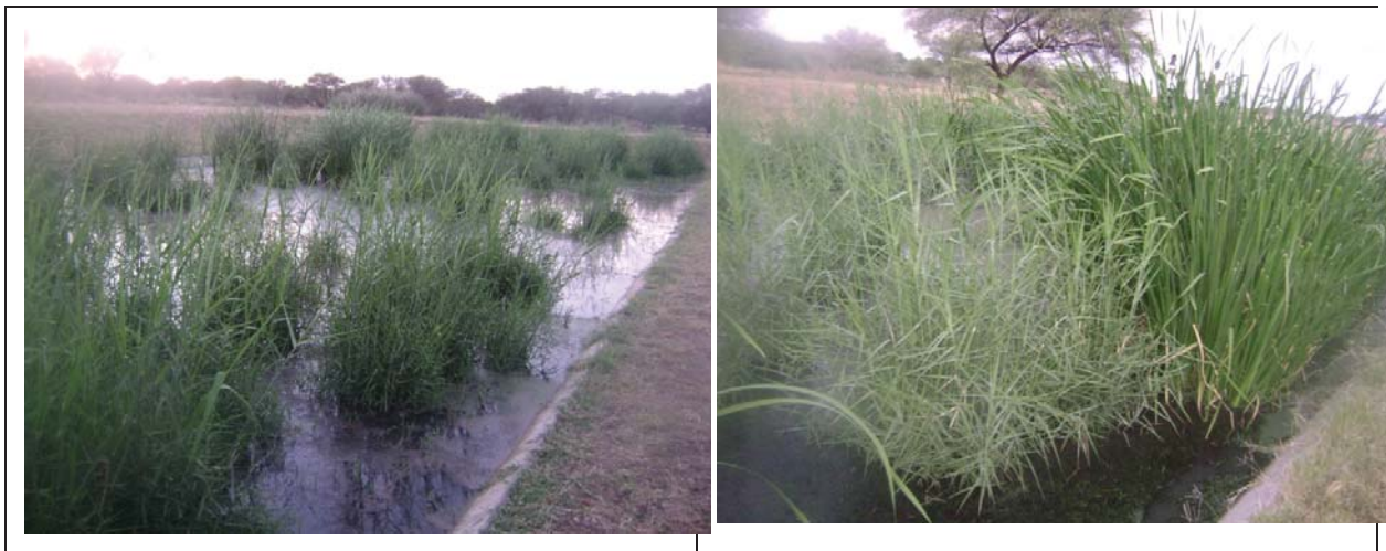
Figure 11: HSSFCW System at Shinyanga Prison
