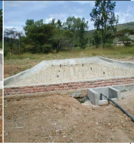
Plate 4c: CW built of burnt bricks In Iringa, Tanzania
