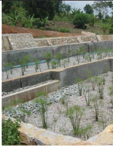
Plate 4a: CW built of stone At Seeta School, Uganda
