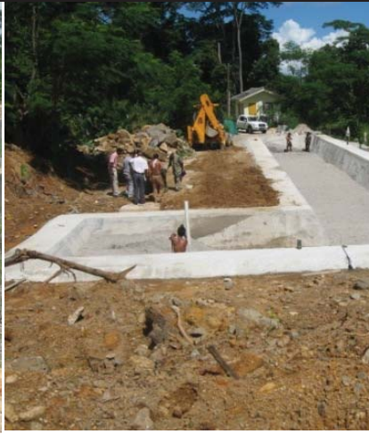
Plate 4b: CW built of concrete In Mahe, Seychelles
